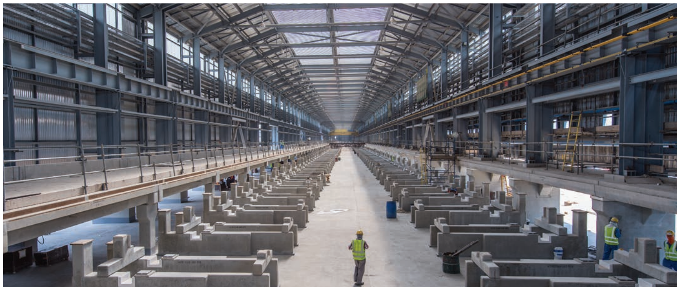
Pot room under construction
