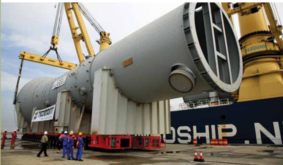
TOP & ABOVE: GIANT COMPONENTS OF THE PETRORABIGH JOINT VENTURE PROJECT ARRIVE BY SHIP AND ARE TRANSPORTED TO THE NEARBY CONSTRUCTION SITE ON MULTI-WHEELED VEHICLES. THE FACILITY, WHEN COMPLETED, IS DESIGNED TO PRODUCE APPROXIMATELY 1.3 MILLION TONS OF ETHYLENE AND 900,000 TONS OF PROPYLENE PER YEAR, PLUS 60,000 BPD OF GASOLINE. PETROCHEMICAL UNITS WILL CONVERT ALL OF THE OLEFIN PRODUCTION TO DOWNSTREAM PRODUCTS.
