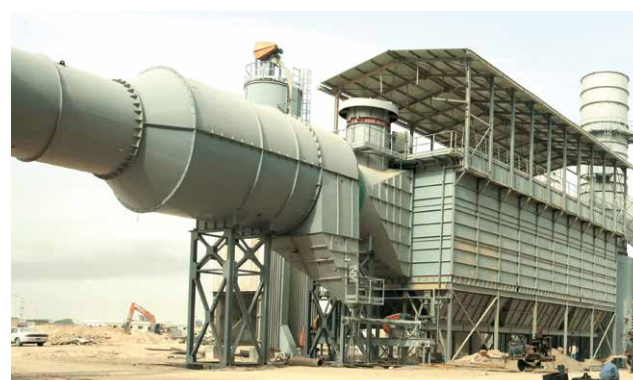
De-dusting System, Al Tanmiya Steel Plant, Iraq
