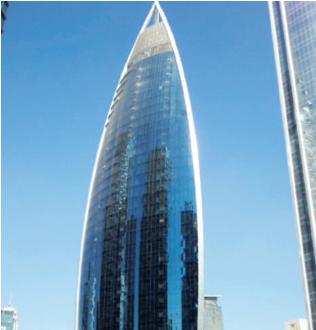
WOQOD Tower in Al Dafna area
