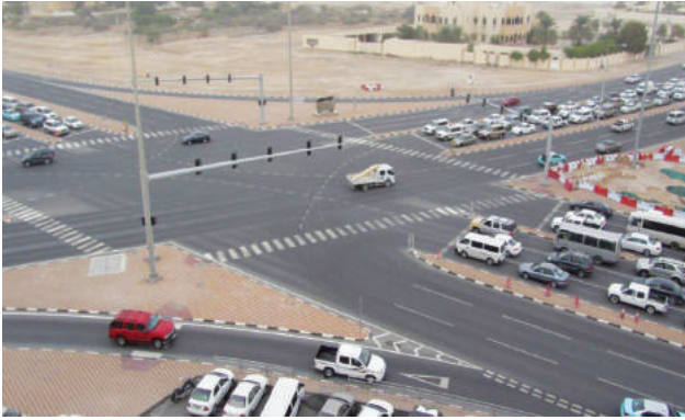
Use of polymer in Doha main streets
