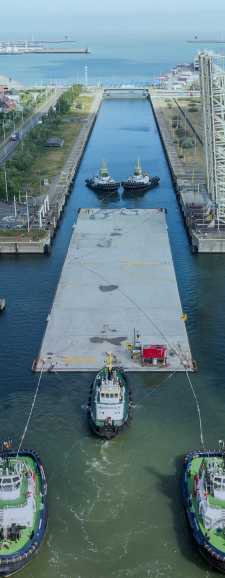
Scheldt Tunnel (Belgium)
