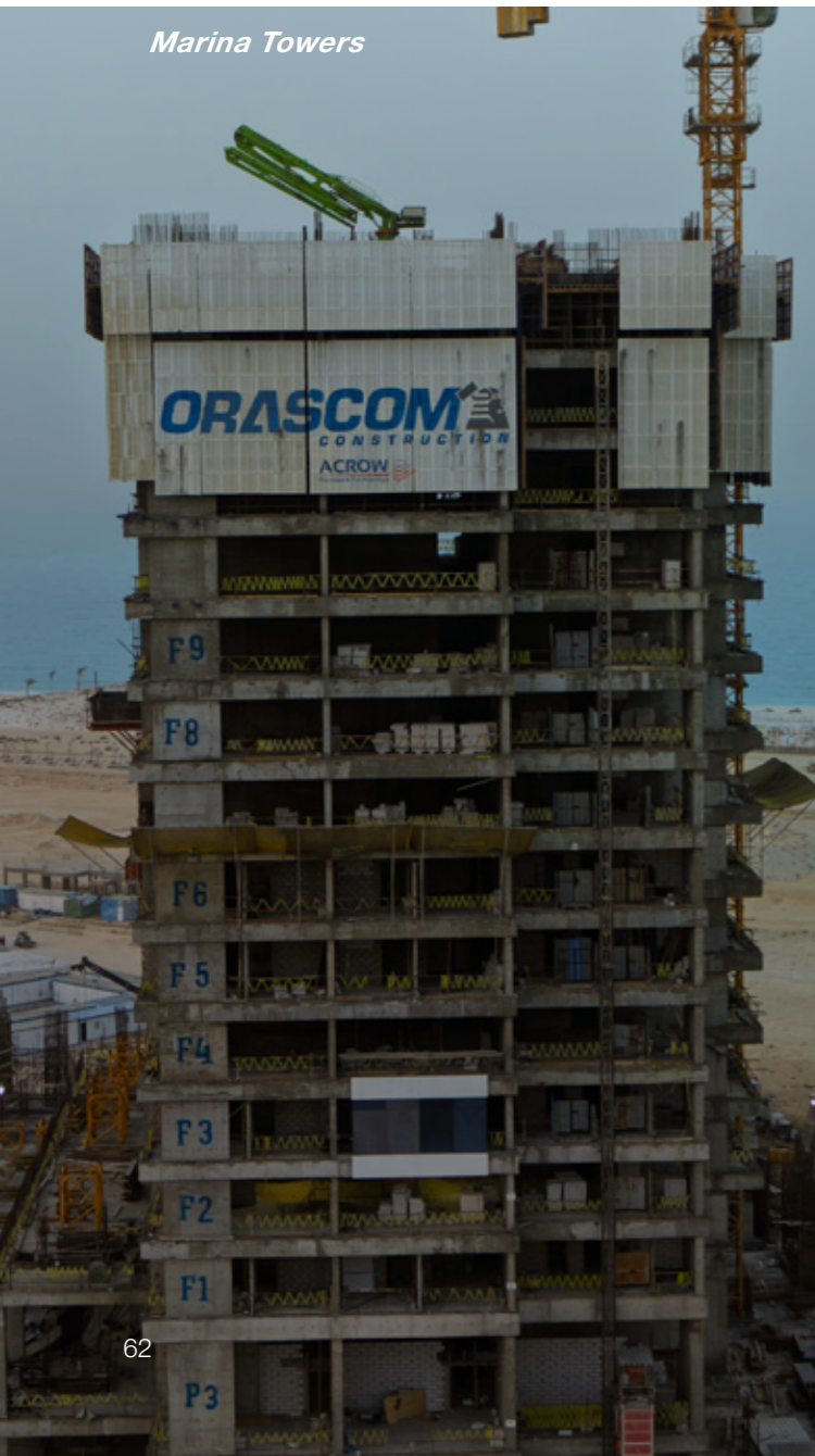
New Alamein High-Rise Towers
