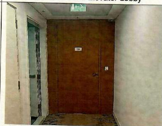
Typical View of Apartments- Unit 201 (sample unit)
