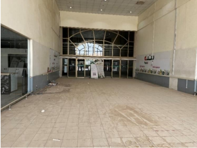
Source: JLL Inspection 2022
