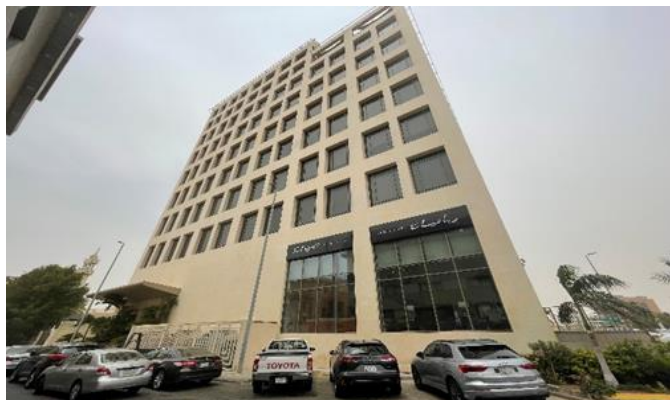
Source: JLL Inspection 2022
