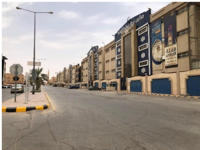
Source: JLL Inspection 2022
