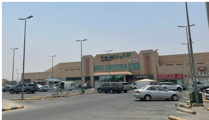
Source: JLL Inspection 2022
