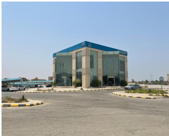
Source: JLL Inspection 2022
