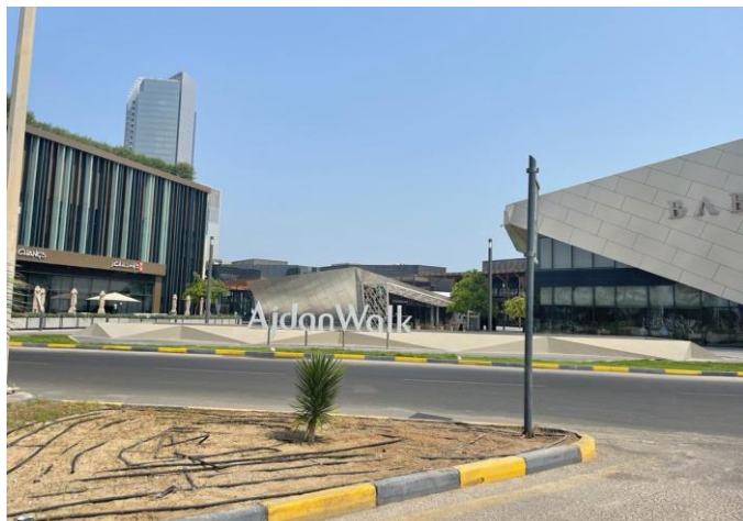
Source: JLL Inspection 2022
