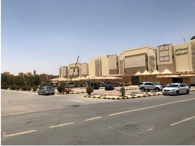
Source: JLL Inspection 2022
