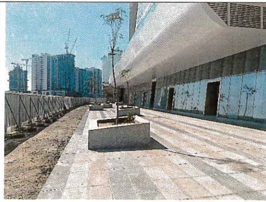
View of Walkway-waterfront area
