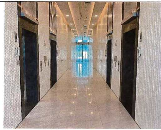
View of Ground Elevator Lobby
