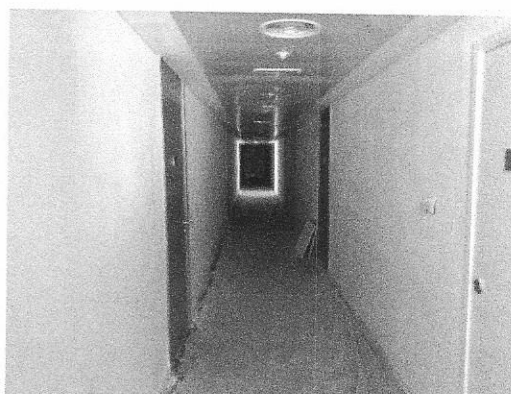
Common Corridor – 2 nd Level
