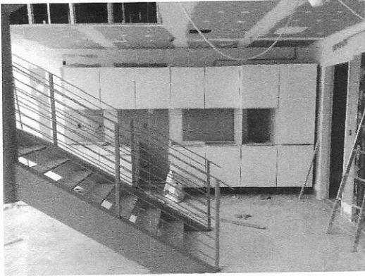
Integrated living/dining / staircase – loft unit
