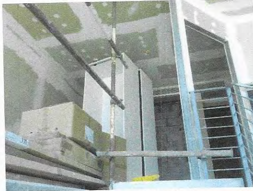
Loft – upper level
