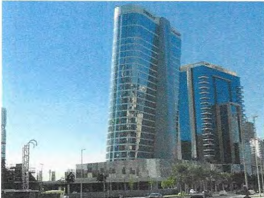
Subject Tower (The Pad) front elevation
