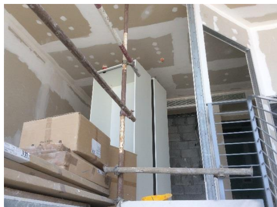
Loft – upper level
