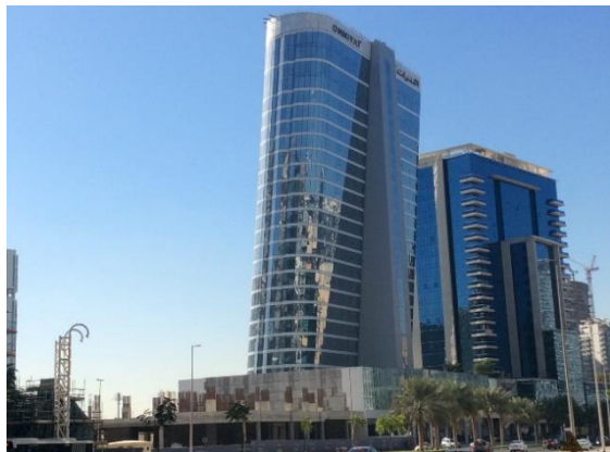
Subject Tower (The Pad) front elevation
