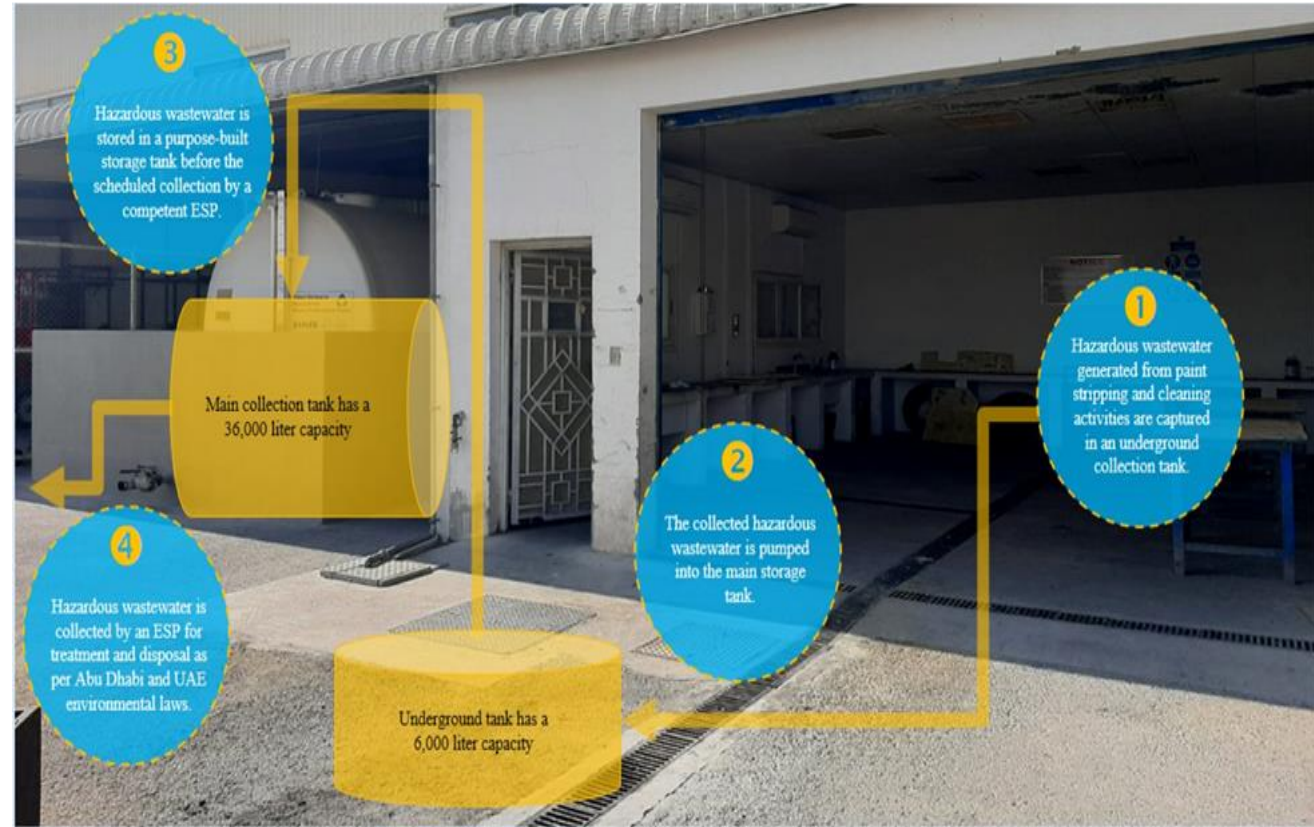
Process workflow – hazardous wastewater generation, storage and collection
