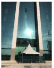
Olaya Tower 1 is an eight-storey with annex and two-level basement parking, mainly built of reinforced concrete structure. We were not able to inspect the offices areas due to on-going renovation at the time of inspection; however, external building finishes consist of glass curtain and aluminium cladding external façade, concrete exterior wall, glass on aluminium frame windows and main entrance door, marble elevator lobby wall, painted interior lobby wall and ceiling.
