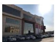
Building finishes consist of glass and aluminum cladding façade and concrete exterior wall, painted and marble tiles interior wall, marble/granite tiles flooring, painted suspended ceiling and some vacant office spaces with bare ceiling, wooden interior doors and glass main entrance doors.
