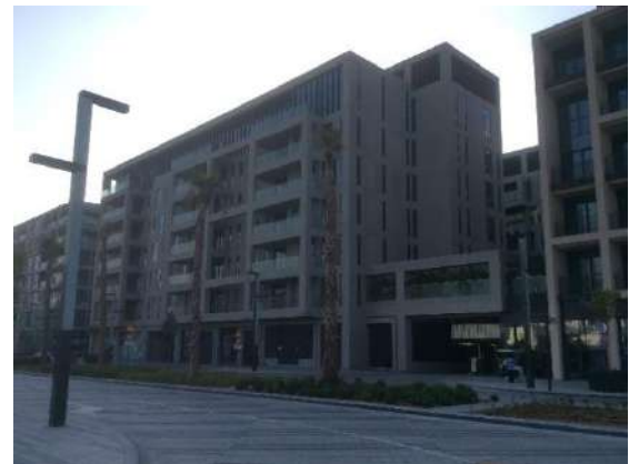
Subject Property – Rear Elevation
