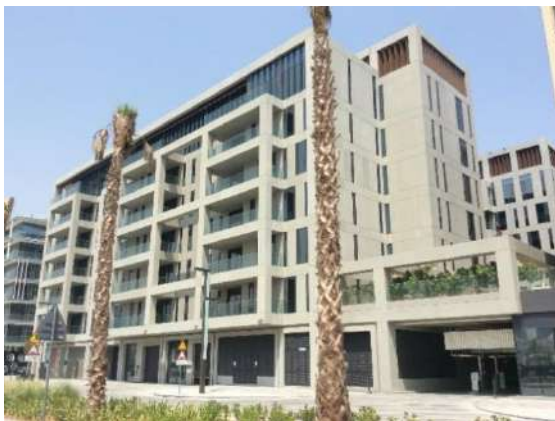
Subject Property – Rear Elevation
