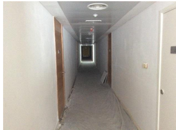
Common Corridor – 2 nd Level
