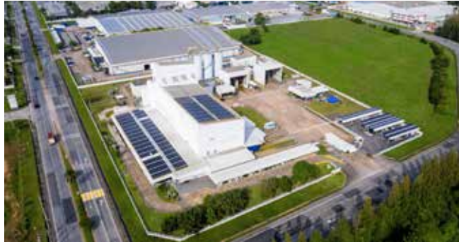
SABIC's sustainability initiatives in Asia also involve reducing the carbon footprint of its operations. At Rayong, Thailand, for example, a 2MW on-site solar farm project generates around a quarter of the plant's energy needs.
