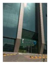
Olaya Tower 1 is an eight-storey with annex and two-level basement parking, mainly built of reinforced concrete structure. We were not able to inspect the offices areas due to on-going renovation at the time of inspection; however, external building finishes consist of glass curtain and aluminium cladding external façade, concrete exterior wall, glass on aluminium frame windows and main entrance door, marble elevator lobby wall, painted interior lobby wall and ceiling.
