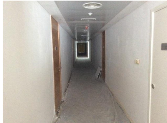
Common Corridor – 2 nd Level
