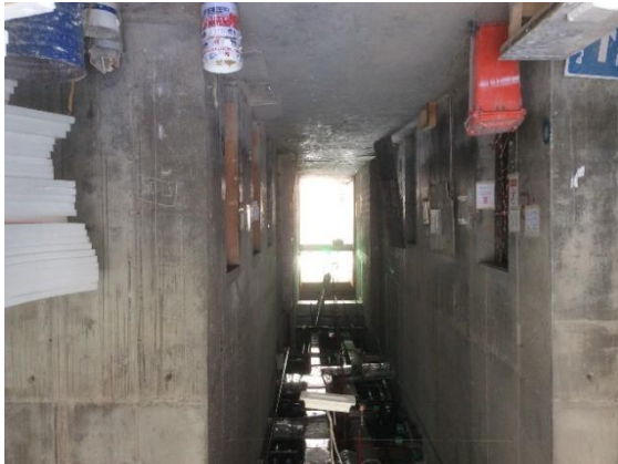
The Pad Tower – Main lobby
