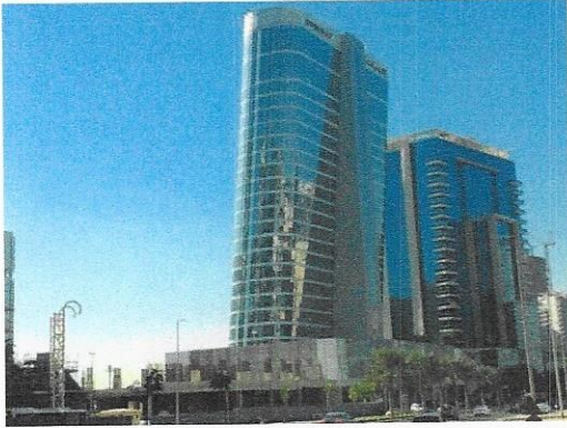
Subject Tower (The Pad) front elevation
