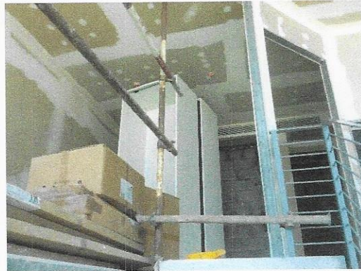
Loft – upper level
