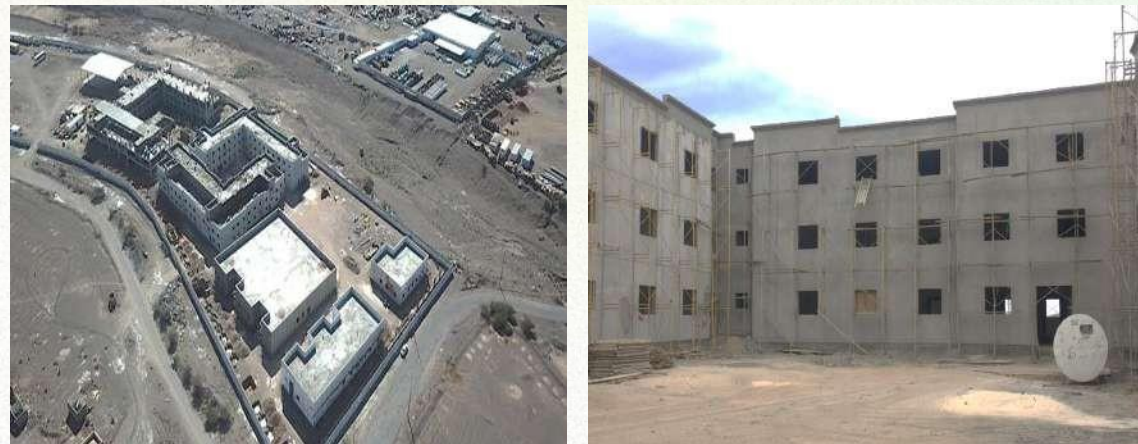
Project Current State
