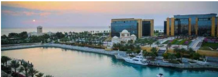
The largest integrated leisure & hospitality district in KSA on the Red Sea
