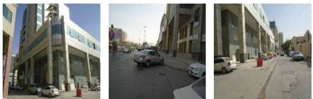
Property No. 4 – Commercial/offices, King Fahd Road, Al Mohammadeya, Riyadh.
