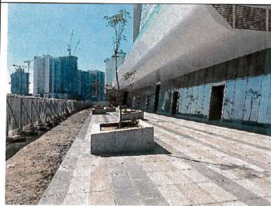
View of Walkway-waterfront area
